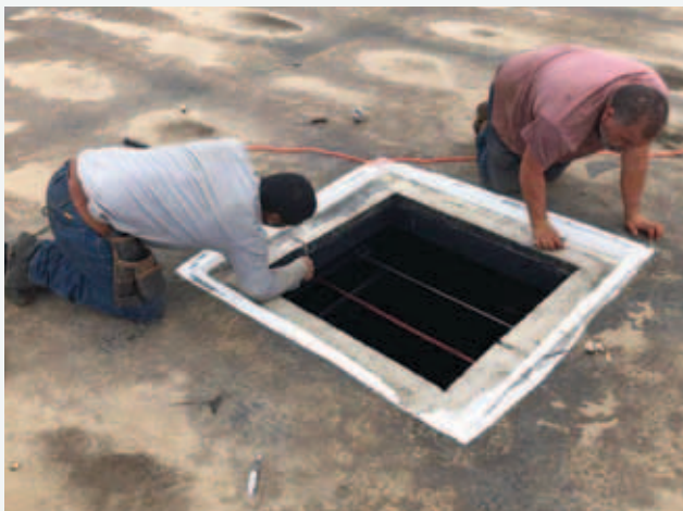
Filling in where a skylight once was
