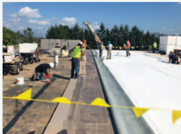
New TPO roof covering going down
