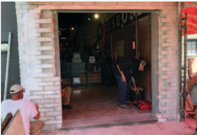
Bob Adams Masonry begins to make an opening in the wall
